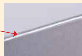
Particular on the fillet welding. It is possible to notice the remarkable degree of finishing and the high welding precision
